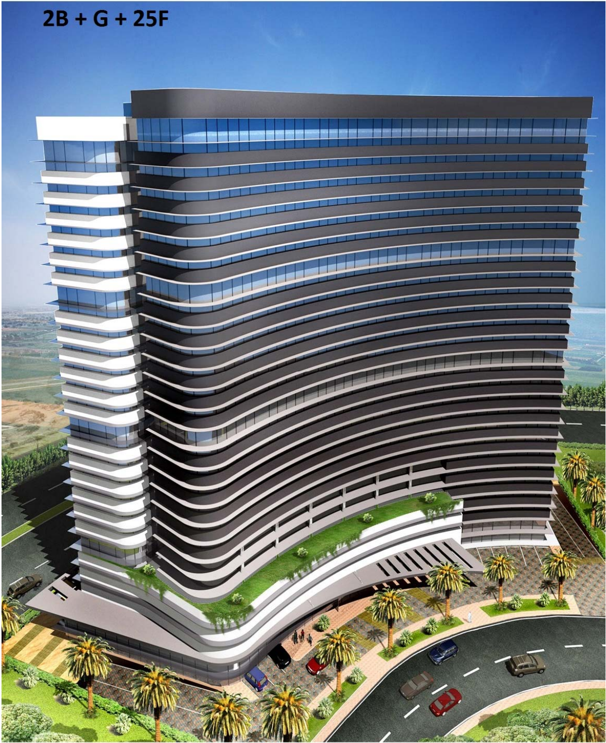
Curve Hotel Tower at Dafna : 2B+G+25 Floors
